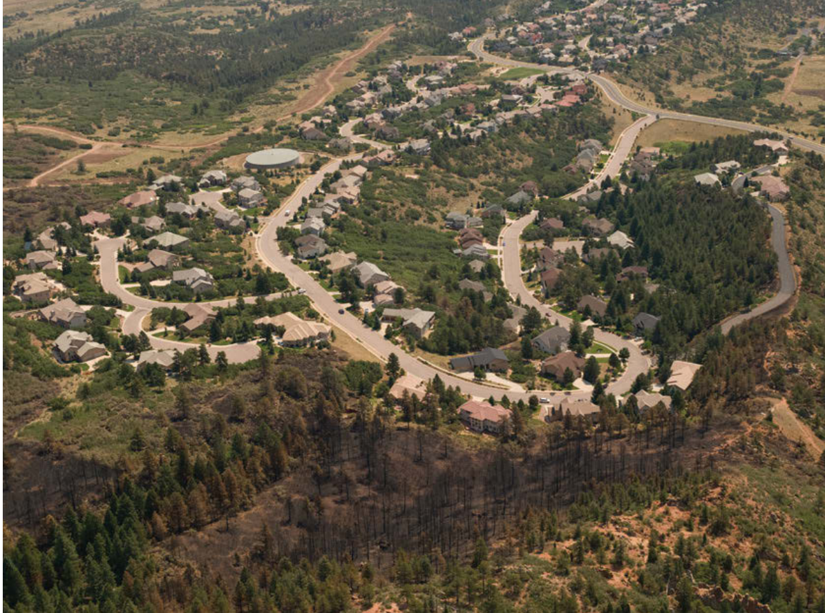
Waldo Canyon Fire, Colorado Springs, CO, July, 2012. Aerial photograph of the wildland-urban interface. Note the fire scars (brown/gray color) reaching the limits of the neighborhood, and the roads and water storage tank potentially threatened by wildfire. Photo by Kari Greer, used with permission.
